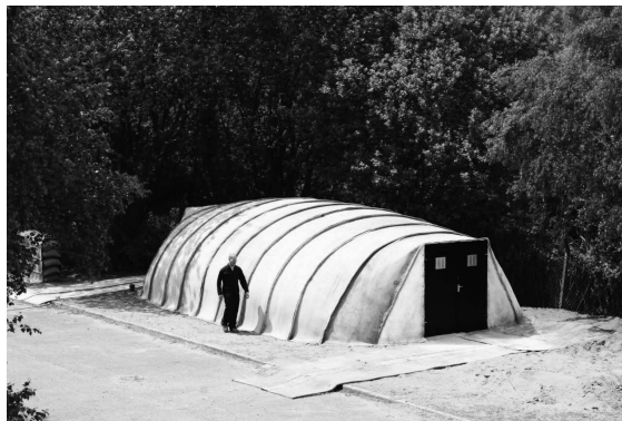
Figure 2. Concrete Canvas was originally designed for shelters
