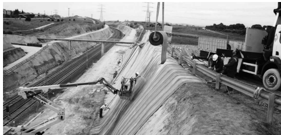
Figure 1. Concrete Canvas used for slope lining
